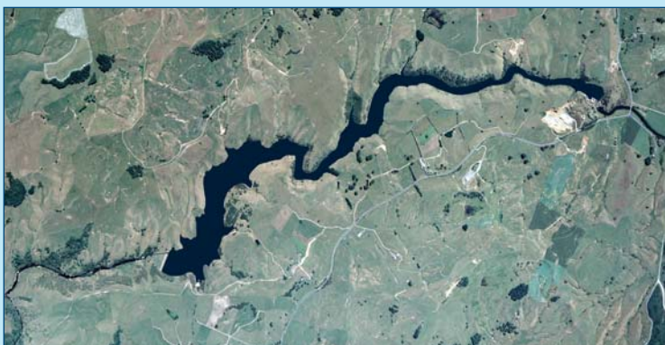
Above: The proposed Mokau Hydro Electric Power Scheme will create a 4.3km lake with a surface area of 50 hectares.
